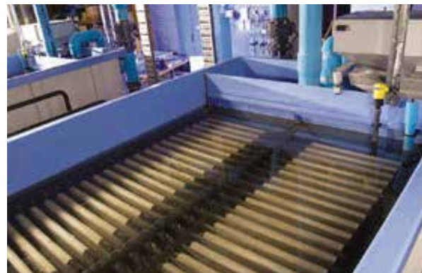
Vacuum DE filters (source: Ian Coombes Ltd)
